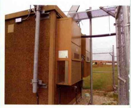
A prefabricated building can have all the HVAC and electrical work installed before the unit is delivered.
