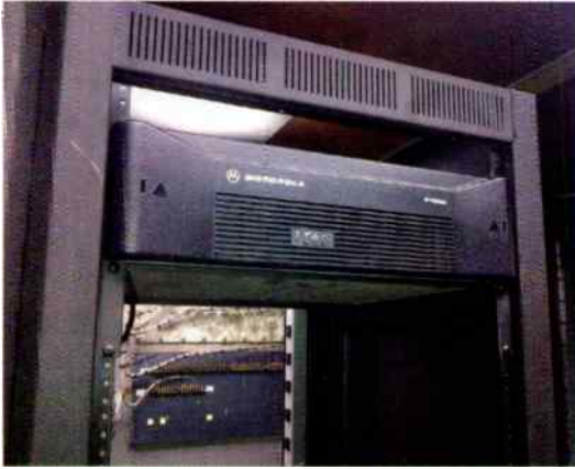
Figure 3. Remote base station transceiver located in the Hollywood Hills above Los Angeles
