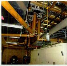
Coaxial switch and transmission line routing for KCBS-FM and KTWV transmitters
