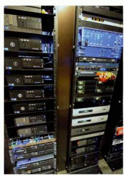
Left rack: Op-x automation and VoxPro PCs; right rack: codecs and AoIP studio engines
