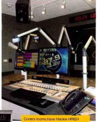
studio monitors, clocks and timers from ESE, Telos VX phones, 360 Systems Instant Replays and a WideOrbit digital media playback system.
