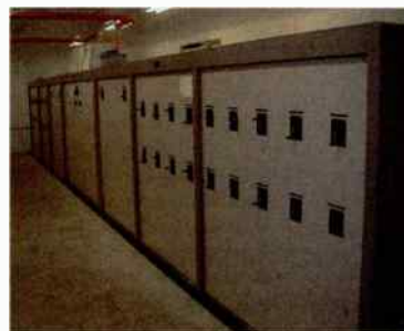
CUSTOM PHASOR INSTALLATION
