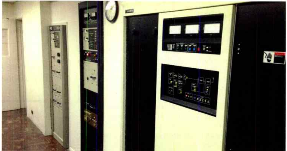
A worthwhile strategy to consider is having two auxiliary transmitters, in addition to the main.
