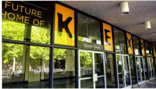
The main entrance already features station branding.
