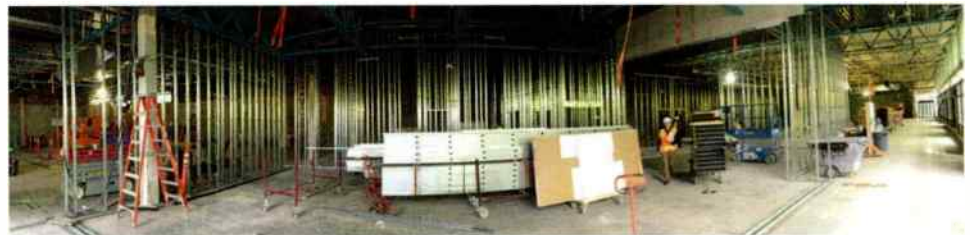
This summer, construction began on the new facility.
