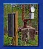
Kintronic Isocoil ISO-170-FM-N for 4-FM station combined antenna feed on AM tower
