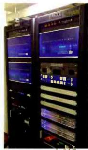
The three-frame 32KD router makes up the heart of the SAS system at Westwood One's Culver City facility.
