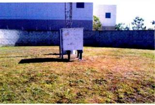
Fig. 1: This is how all AM tower bases should look-free of weeds.
