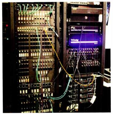
The wiring rack is the central nervous system of the entire facility. This rack includes KVM switches and Cisco switches for the AoIP network, as well as the TV production equipment and PEG channel server.
