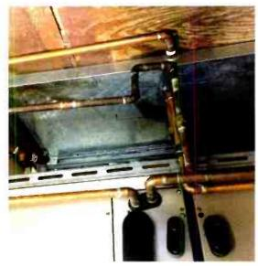
Fig. 2: Keep condensate pans free of debris. This will keep drains clear.
