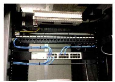
Figure 2: Network Switch, Patch Bay and Krone Block
