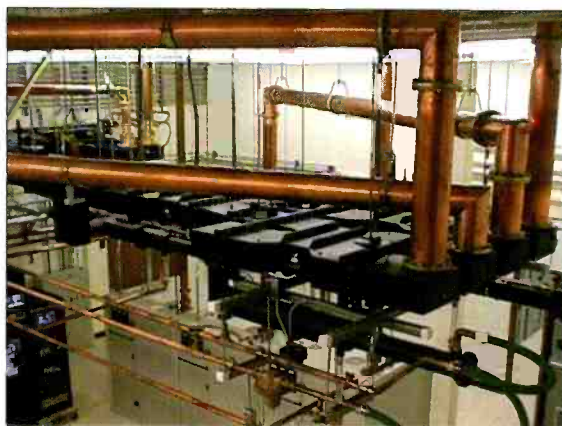
Rigid transmission line (shown above) is often the choice in North America, while semi-flexible line has traditionally been used in Europe and Asia. Photo courtesy Dielectric.
