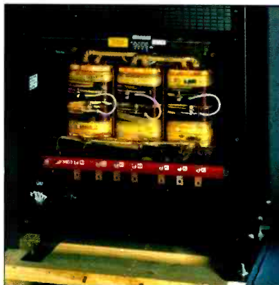
The PowerSmith T-1000 zero sequence impedance transformer offers a practical solution to power quality issues.
