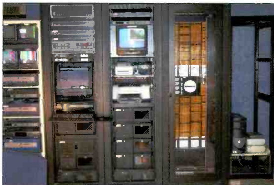
At the heart of the completely tapeless system is a TiltRac hybrid server system, which uses DVD-RAM for archive. The server will act as network-area storage until the new 8TB storage-area network is installed.
