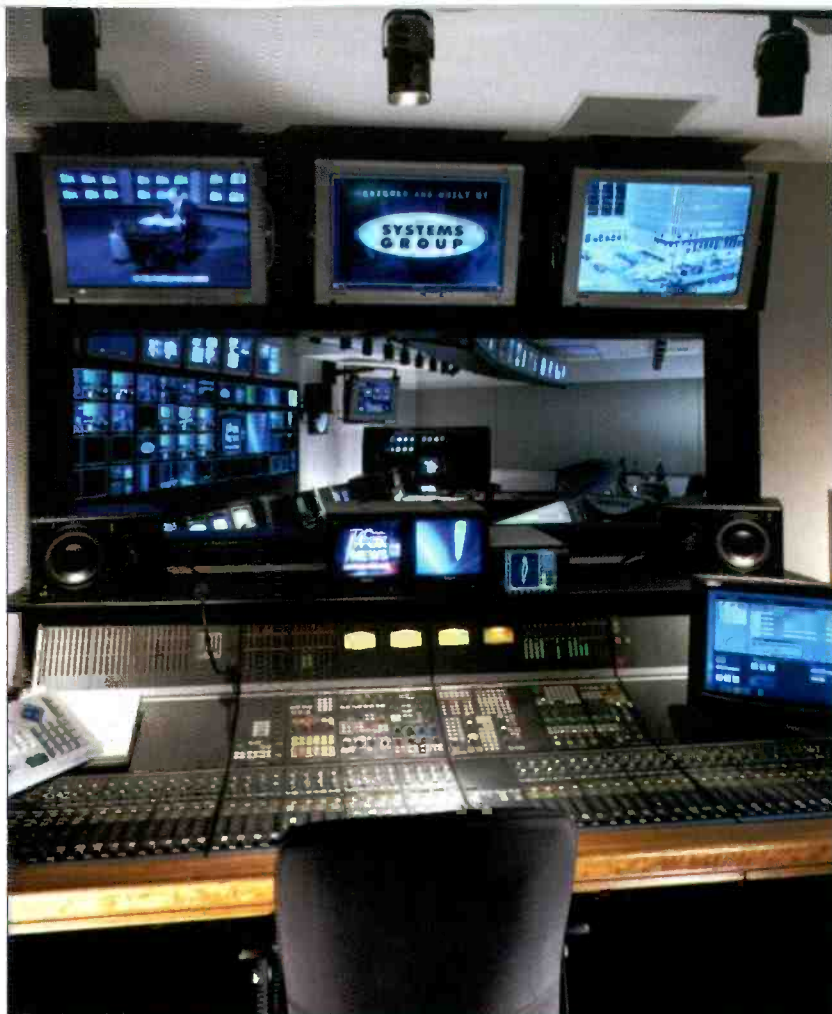
FOX's audio control room overlooks the production control room. The new audio room is designed around a Calrec Sigma 100 digital audio console.
