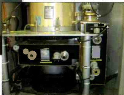
The primary and secondary output cavities of the IOT are air-cooled and should be kept clean to keep the high-voltage arc detector working.
