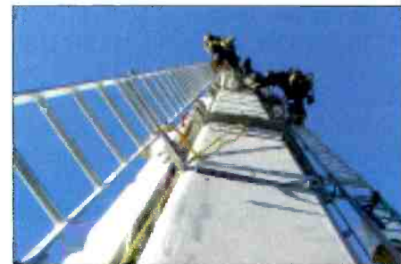
Dual broadband panel arrays from RFS provide sculpted digital/analog signals for four Los Angeles broadcasters at Mount Wilson.
