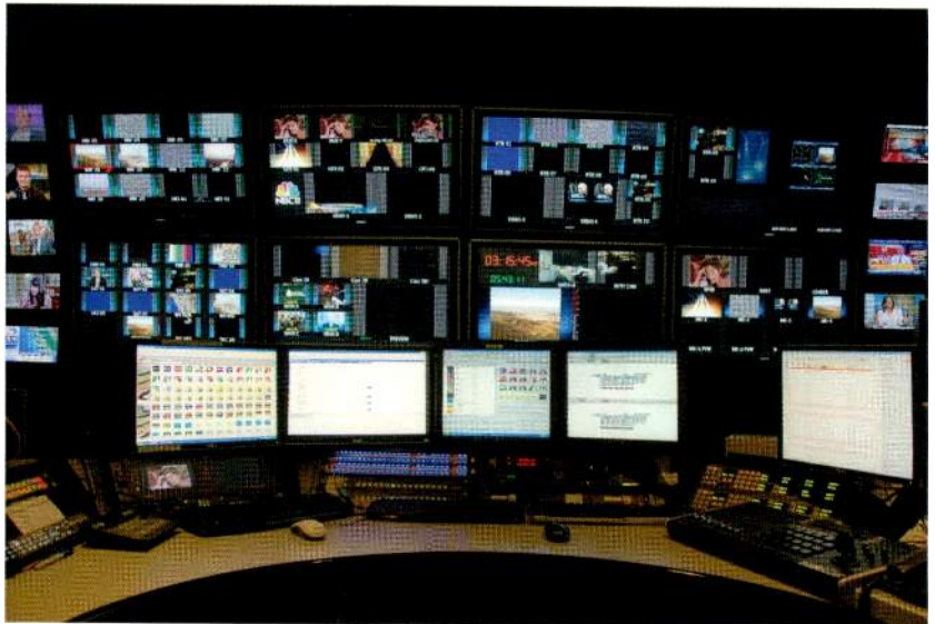
The control room at KNTV in San Jose, CA, features a Ross Video OverDrive automated production control system.
