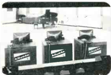
Control-room view of three A-7 Systems used for 3-channel PLAYBACK monitoring at United Recording Studios, Hollywood.
