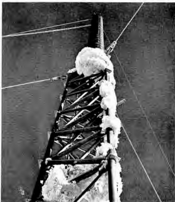
Fig. 1. A heavily-iced tower with fiberglass-covered FM antenna.
