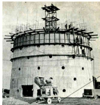
Scaffold and forms for one 7½' section.
