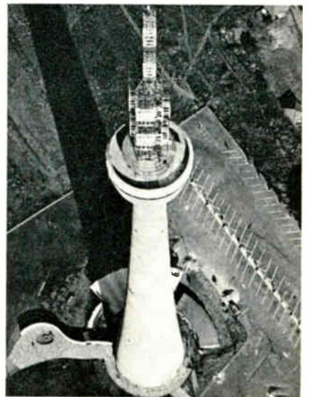
Aerial view of the concrete FM tower.
