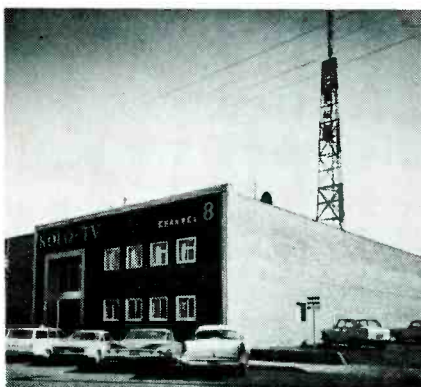
Reno terminal of the microwave system.
