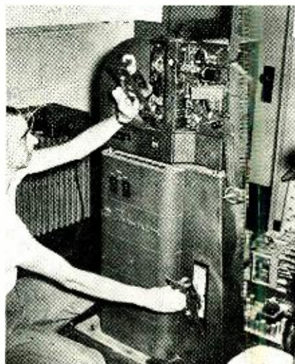
Fig. 4. Film projector has spare lamp in base; manual changeover required.
