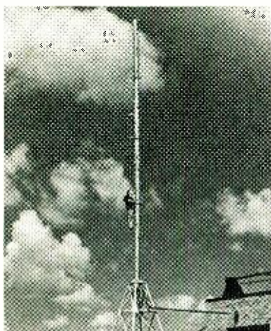
Fig. 4. A four-bay UHF helical antenna.
