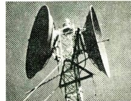
Microwave dishes at one of two stations relaying network programs to WTWO.
