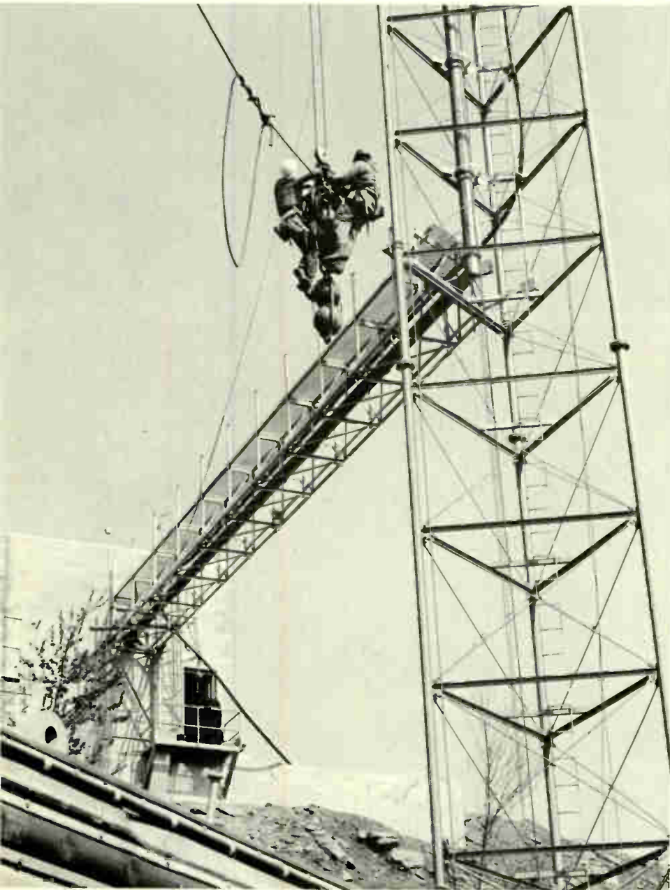
Fig. 9 Antenna tower bridge assembly.
