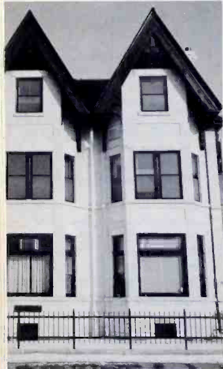
Fig. 1 Exterior of Eastern Sound's studio in Toronto. Renovation did not disturb old building exterior.
