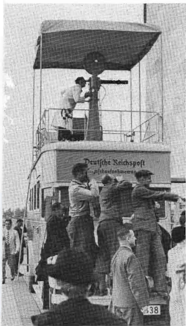
One of two mobile TV vans with a film camera on the roof that fed the film processor and optical disc scanner inside. Pictures were in monochrome, non-interlaced, and had 180 lines at 25 frames.
