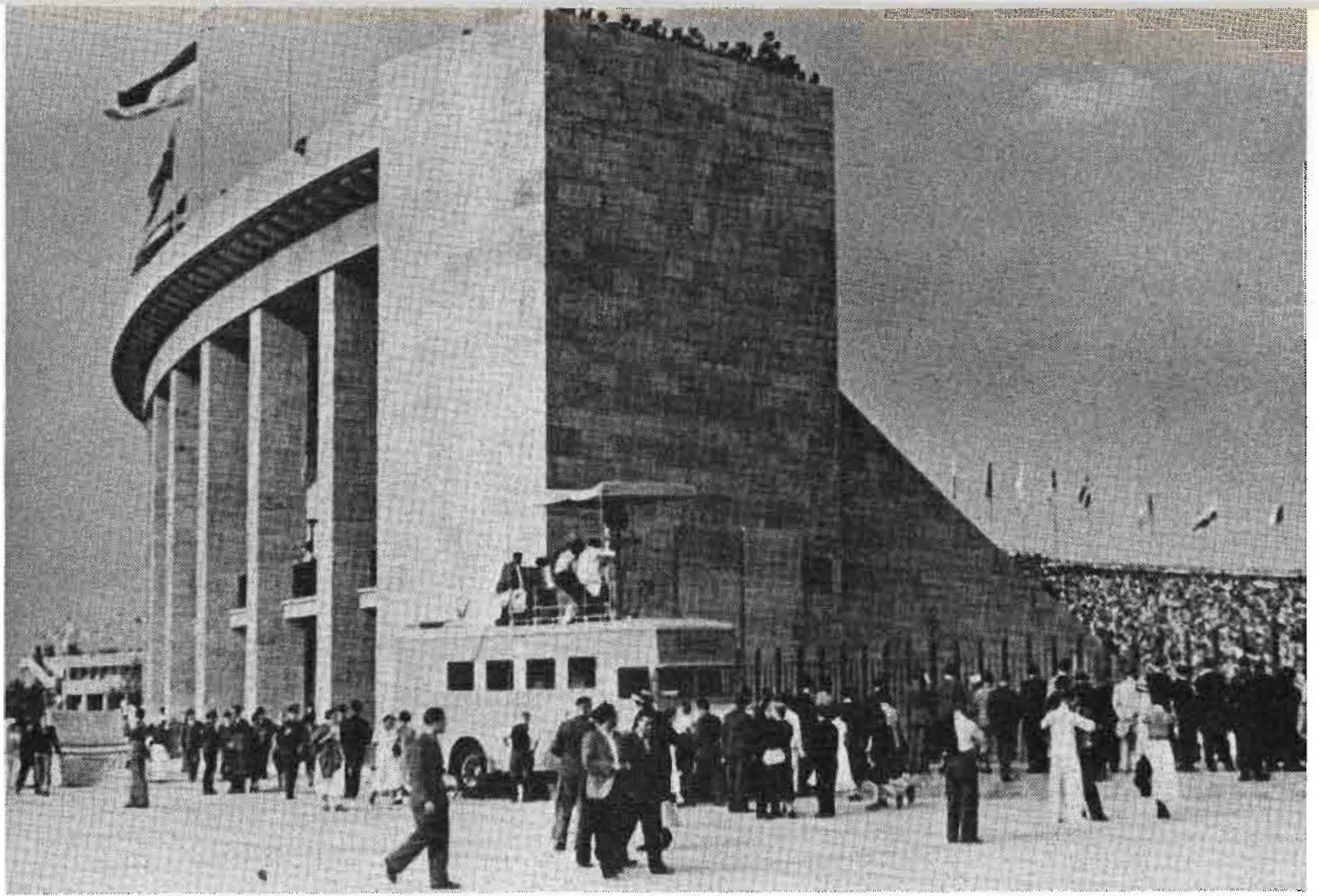
Parked near the Marathon gate of the main Olympic stadium, the Reichpost's mobile van, with the intermediate film system, was restricted in position and coverage.
