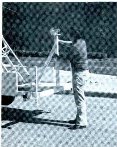
...the tower hoisted,...
