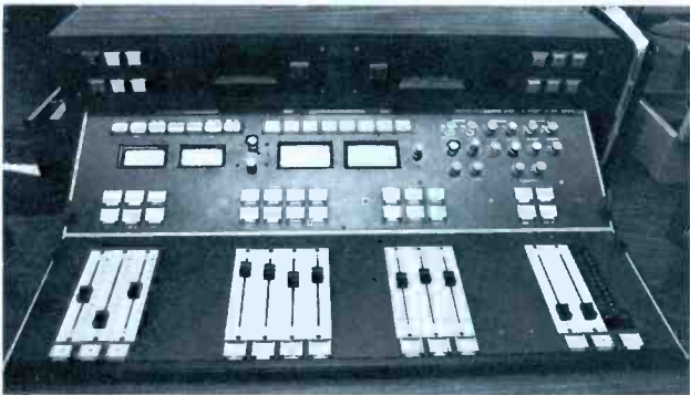
Figure 2 The studio 8A console close-up view reflects maximum simplicity in design for the WABC air board.
