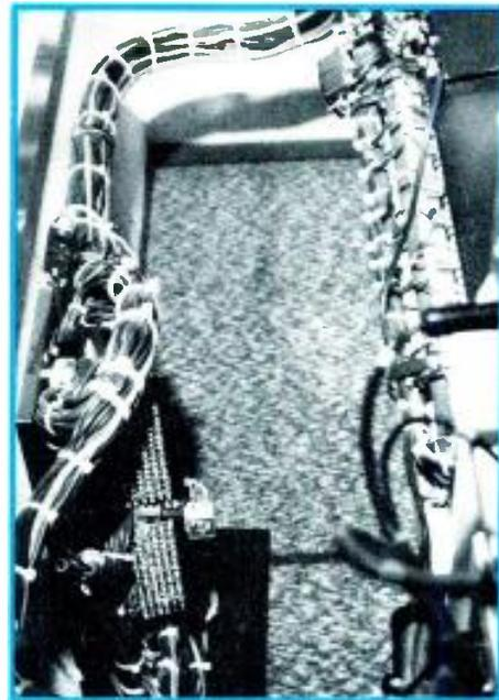
An access path of at least 18 inches should be left behind the control room equipment to allow servicing.
