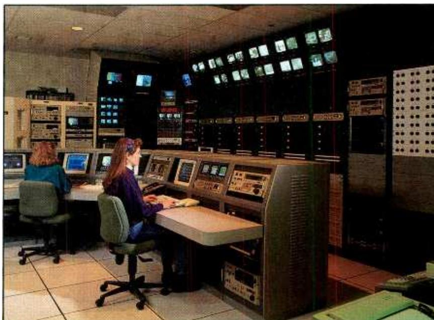
*StarNet control room in West Chester, PA, monitors and retransmits all ad-supported cable network cue tones and deploys an MPEG digital uplink to send commercials to affiliates for storage and playback.*
