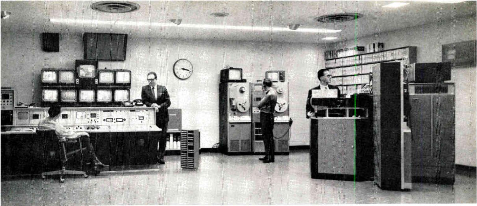
VTRs and film island are located in close proximity to the master control console. In view of master control and the entire areas is the transmitter, located to the left. The additional space in this area may be used for another film island, VTRs, and color camera power supplies.
