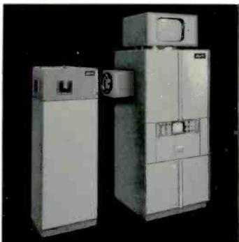
Norelco's PCM-800 Multiplexer is designed specifically for the PCF-701 Film Camera. Slides can be supered over film on the same film island for the first time in color TV.
