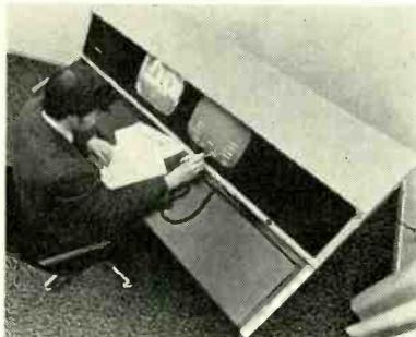
CMX 600 that allows either video tape or film to be edited electronically using only a light pen to make a finished production. High speed minicomputers perform every tedious chore, remember editing decisions, and accomplish the assembly.
