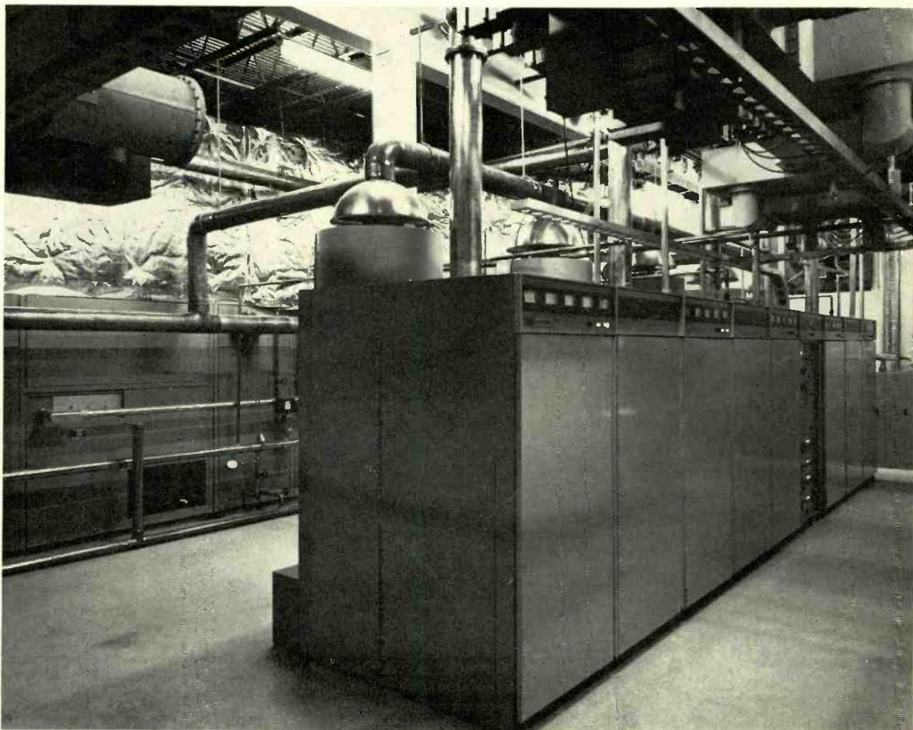
**View of the "World's Most Powerful TV Transmitter,"** a 220-kW Gates Model BT-220U, installed at WDC-TV (UHF Channel 20), Washington, D.C. Station signed on-the-air March 16, 1971. It may also be the world's longest—nine cabinets take up 25 feet. Unit draws one million watts.
