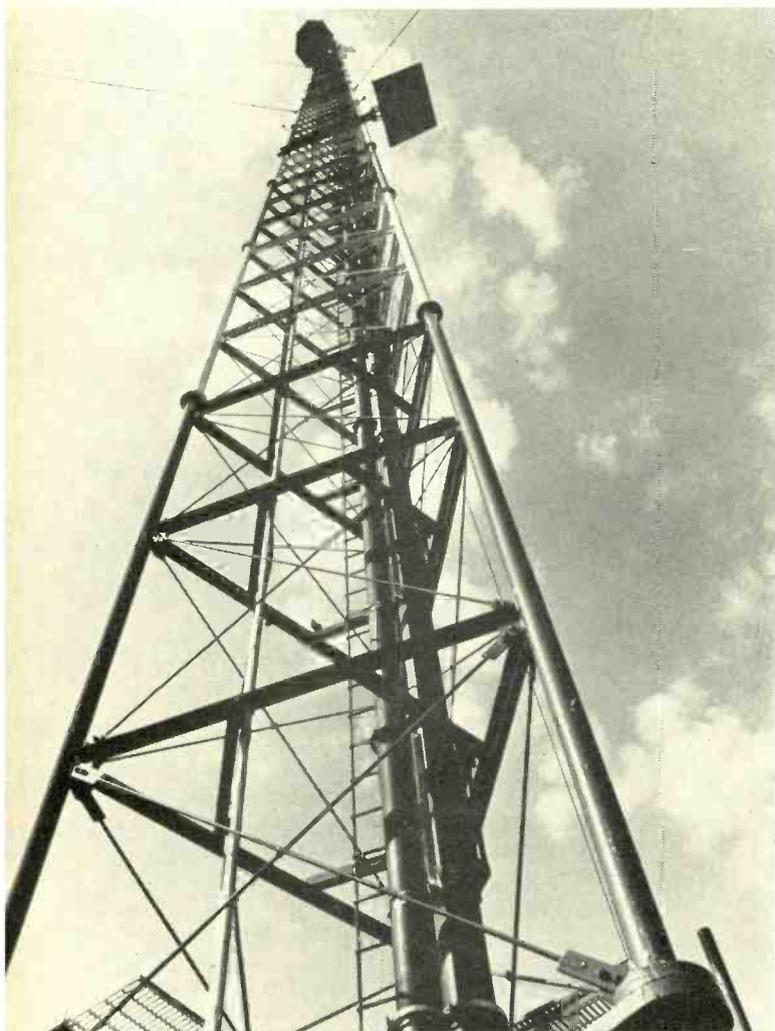
To increase power output from 60 kW to 120 kW, Channel 61, Cleveland, is replacing the 6- $\frac{1}{8}$ -in. coaxial transmission line shown here with a new 6- $\frac{1}{8}$ -in. line using "Freon" HFE coaxial cable gas. The HFE line means an increase in power output with no additional increase in size or weight and no effect on wind loading of the tower.
