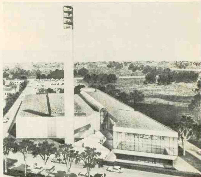
Artist's sketch shows planned KPRC broadcast complex. Striking triangular concrete tower is 180 feet high with microwave STL gear at top. High-vaulted gallery separates TV studios (left) from other facilities.
