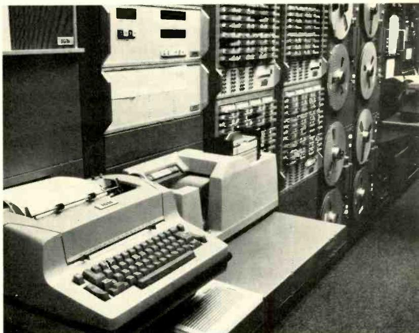
The IGM program automation system at WFIR includes a logging typewriter (foreground) and card reader just past it. Next are two racks of Instacarts and two more of Scully reel-to-reel decks. Finally, a Moseley automatic logger and transmitter remote controls.
