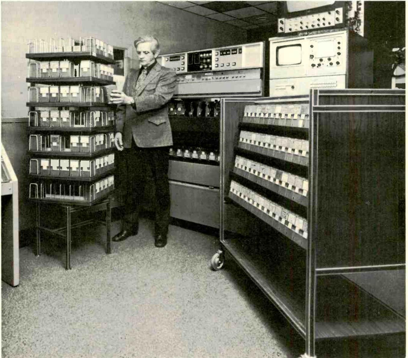
*Illustrated is 7-tier Carrousel (140 cartridge capacity) on a CS-16 Ball Bearing Base, and VTS 16-18 Stand; and CTC-128 Transport Cart (capacity 128 cartridges).*
