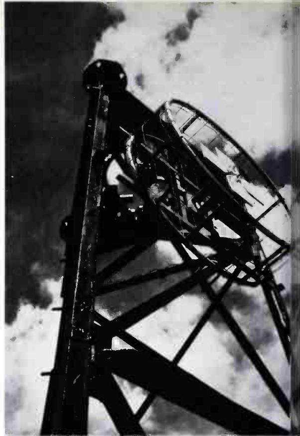
Harris CP antenna has crossed dipoles backed by a cylindrical cavity formed of open wire to reduce wind loading. Rotating field from dipoles excites cavity, which in projection of CP signal at high efficiency.
