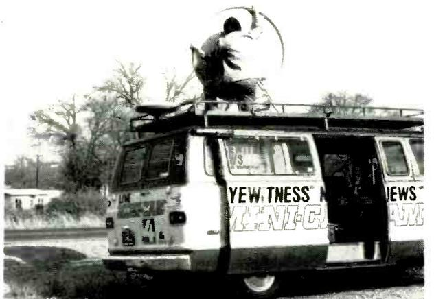
Raising the 2 GHz microwave transmitting dish and aligning it towards the receive site on Sandia Crest.
