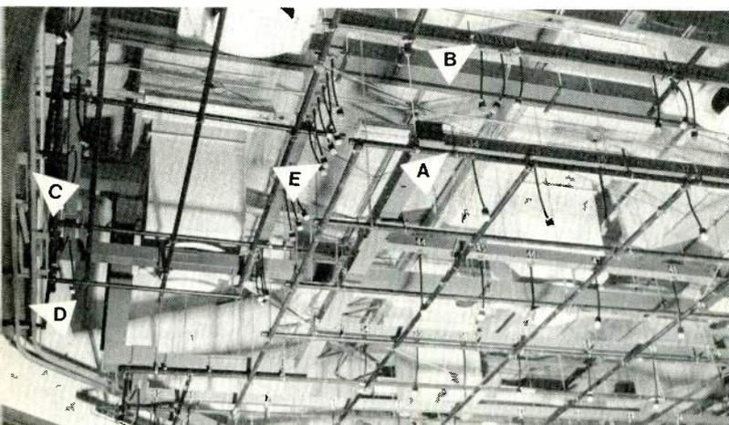
(A) LOWER GRID (B) UPPER GRID (C) CYCLORAMA & DRAPERY TRACKS (D) FLOOR OF PERIPHERAL CATWALK (E) CYCLORAMA LIGHTING OUTLETS (3 color)
