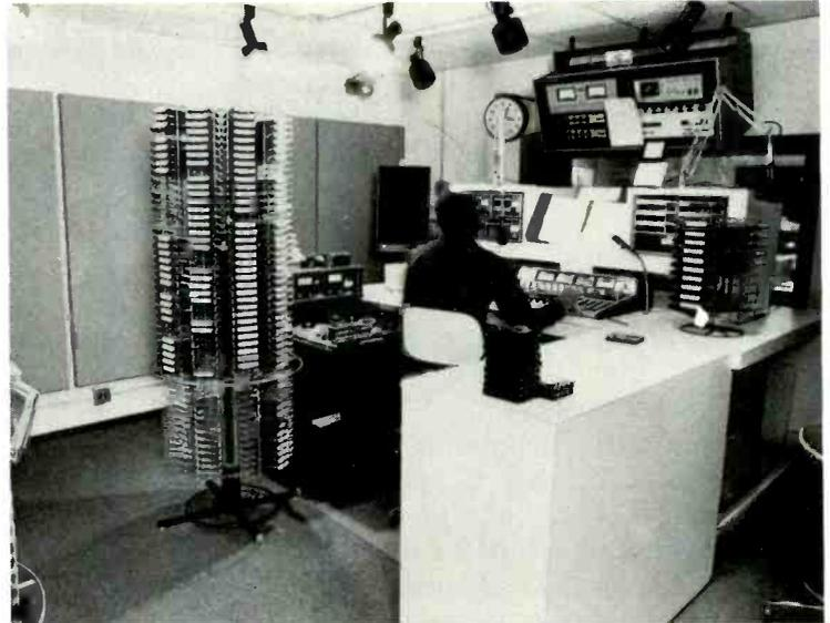
*Control room was redesigned. The entire console is on wheels and plugs into interconnecting cable.*
