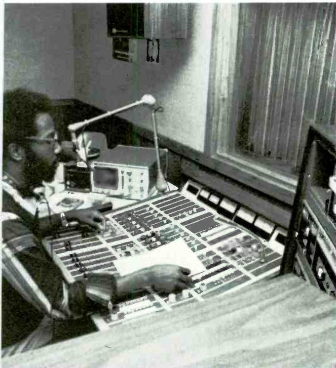
News room has identical McCurdy console, for operator familiarity. Turntables are to left, ITC and MCI machines are at right. Window to main studio is in front of operator
