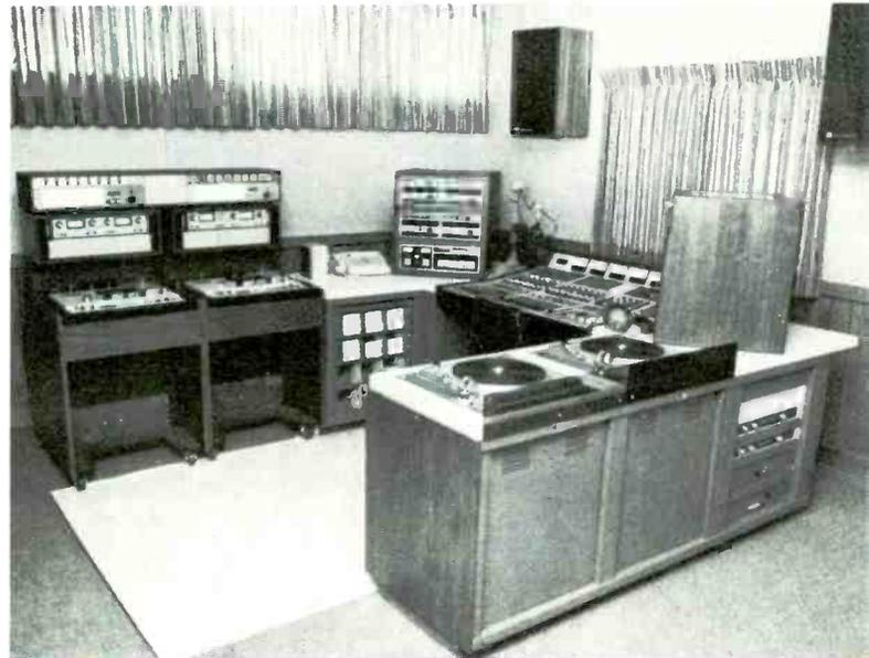
Main on-air studio has Technics turntables at right of McCurdy console, MCI tape machines at left. ITC cart players are uprights at ends of console. All equipment is stereo
