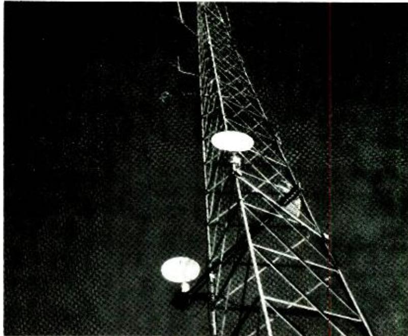
*KRON's installation on Mt. Loma Prieta is the latest to bring on line additional news bureaus. Visible are the steerable dish for pickup of ENG feeds and the fixed 13 GHz return link*
