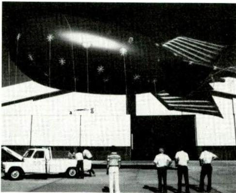
ABC's red "balloon" is 50 feet long and 17 feet in diameter, with a special inflatable fin structure
