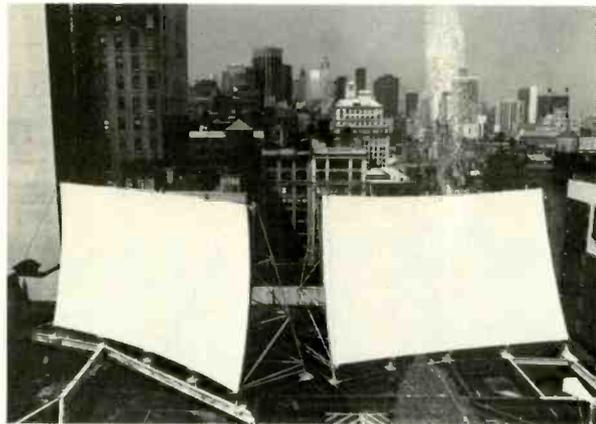
Manhattan Cable TV's twin spherical antennas can receive up to 38 satellites.
