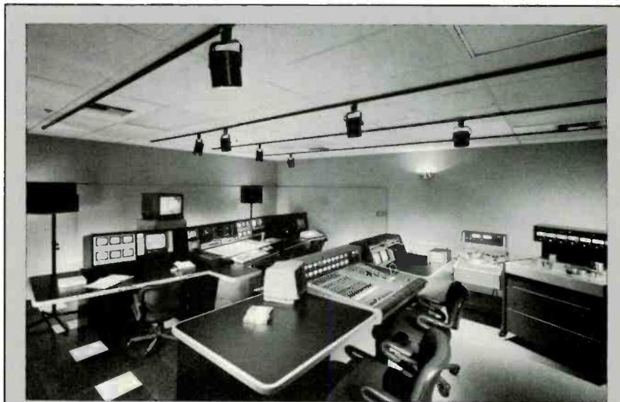
Edit Suite A at Tele-Image's big Dallas facility features a Grass Valley Group 300-3A switcher with E-MEM and E-Disk, Chyron RGU-2 character generator with font and logo compose, a Sony 618 audio console, and Studer A-810 and A-800 synchronous two- and eight-track ATRs.
