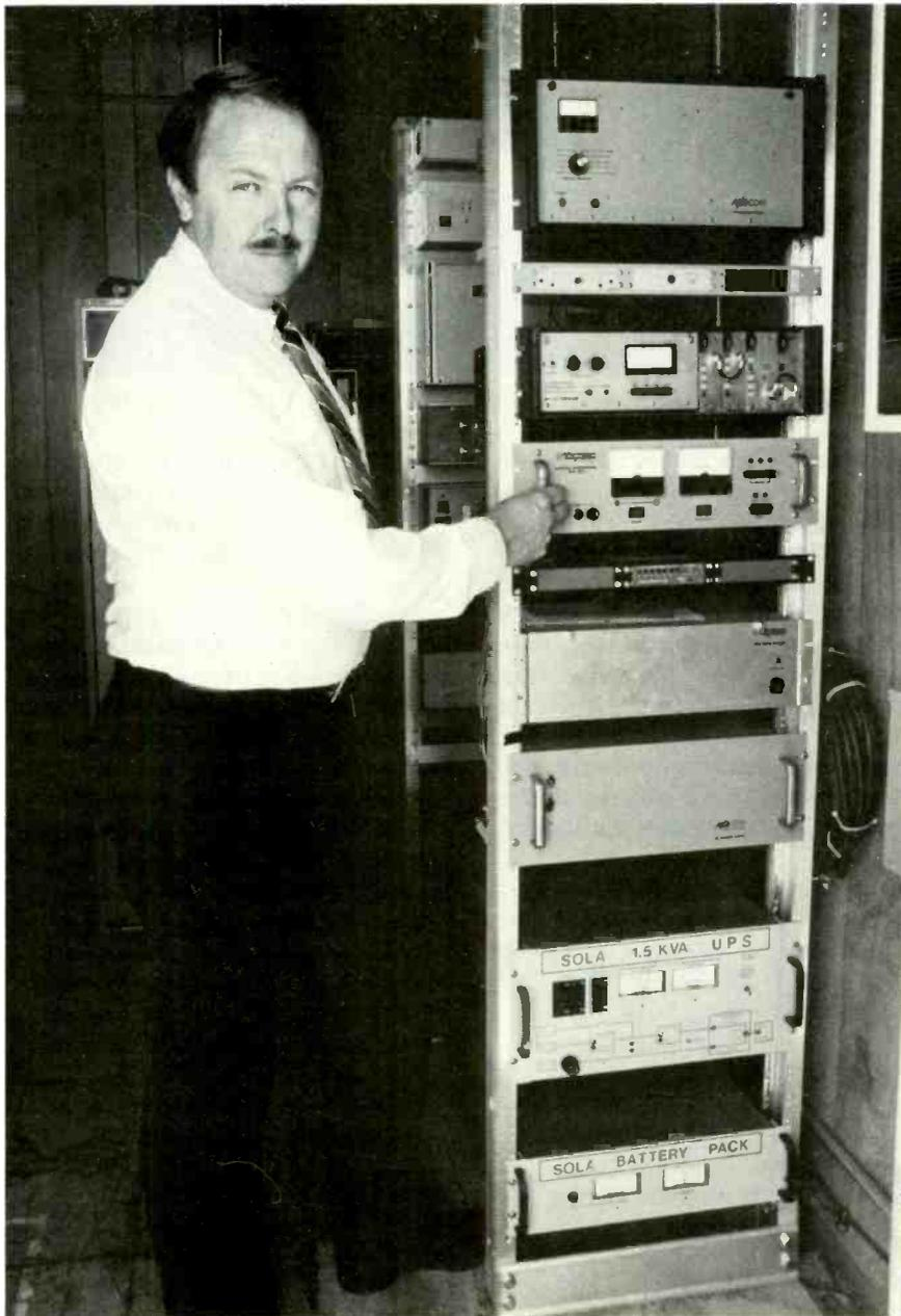
Hutchinson points out the Sola 1.5 kVA UPS installed at the relay site.
