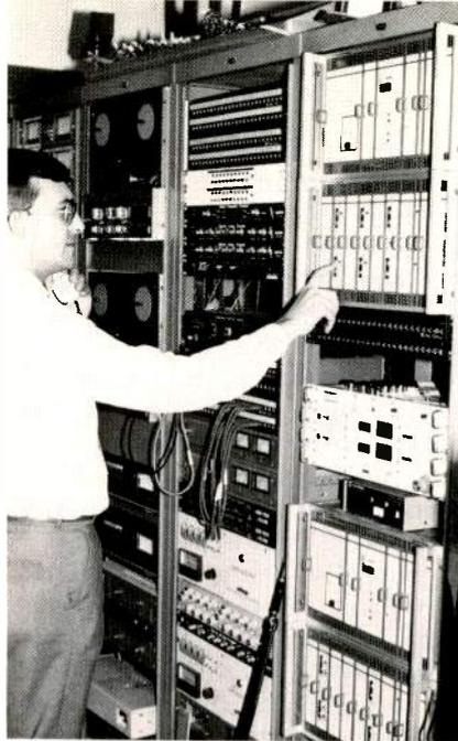
Terry Grieger, chief of engineering for Emmis Broadcasting, in the “wire room” at New York’s WQHT/WFAN. To his left is the station’s backup processing chain consisting of (from bottom) a pair of Orban Optimods, two Audio Prisms, an Eventide Digital Delay, and a CRL Spectral Energy Processor system.
