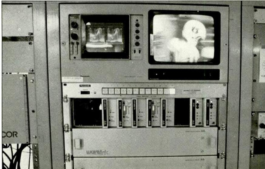
*Fiber optic equipment configuration at the production center in the communications building. The Siecor fiber optic management box/patch panel is just out of frame at the left.*
