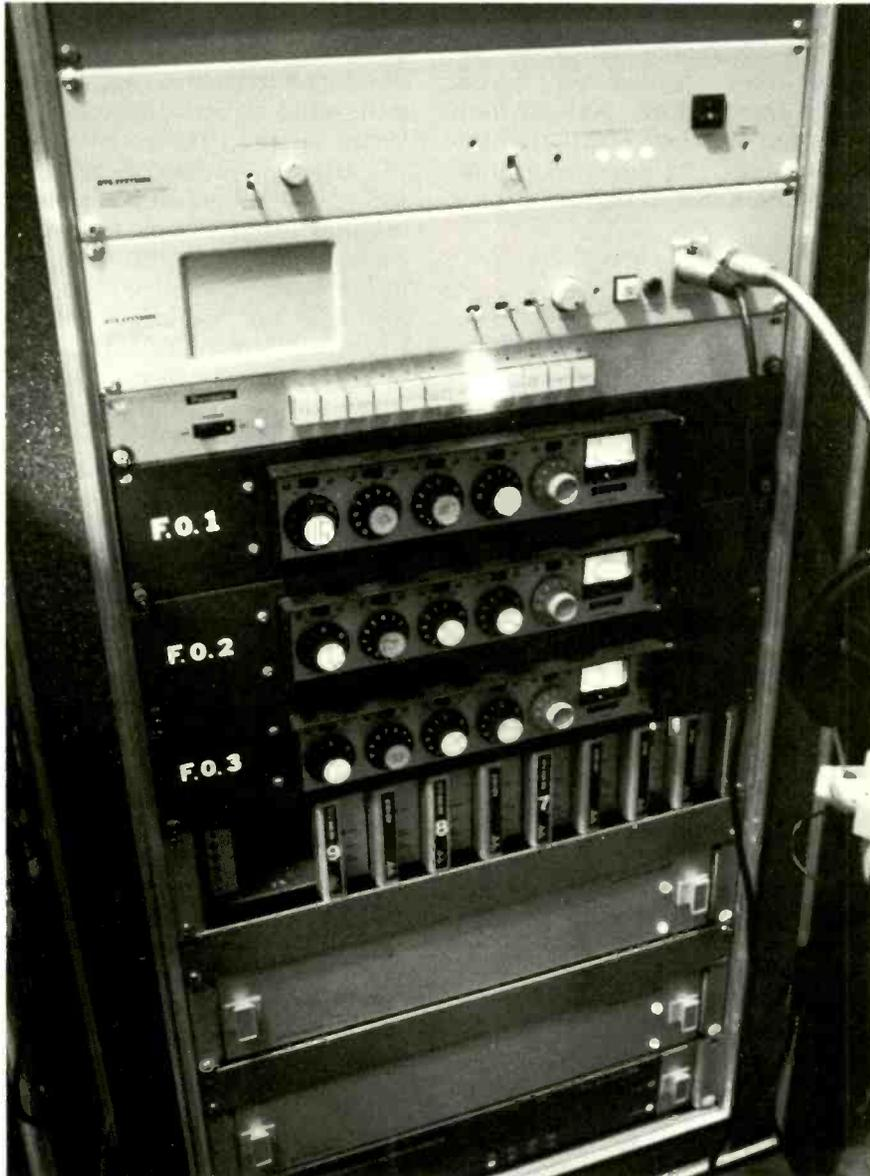
*Remote fiber optic and communication rack. The RTS hardware is at the top. The fiber optic equipment and sync generator are in the lower portion of the rack.*
