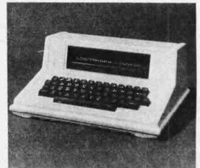
The Transactor I data terminal consists of a single line 32 character gas discharge display with a 5 by 7 dot matrix for easy reading, and a 53 key Teletype style keyboard. It can be attached to almost any computer, with an RS232 or 20 mA current loop interface. Switches allow the user to select the operating mode including 110 to 9600 bps data rate, full or half duplex, even, odd or no parity, five to eight data bits, and one or two stop bits.
