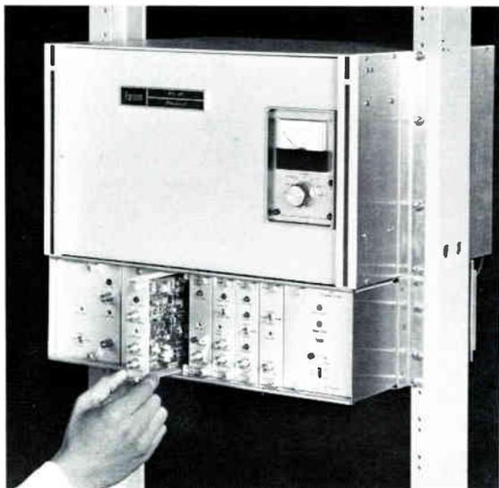
FV4SR Terminal. System shown includes FV4F Receiver and FV45 Baseband Shelf.
