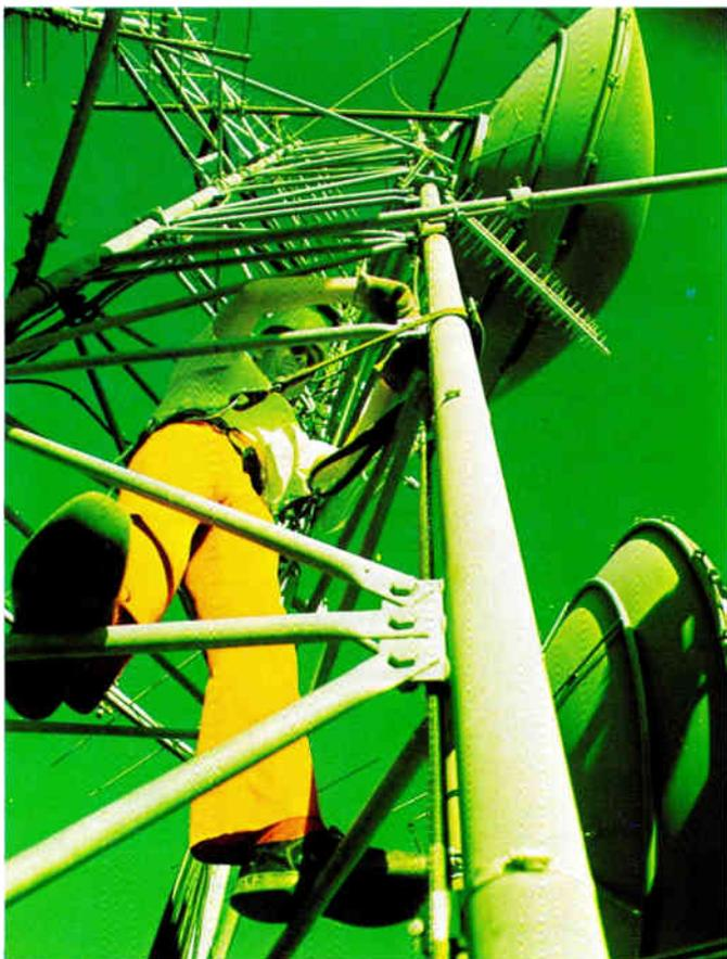
Technician aligns antenna to bring in path signals to receiver site.
