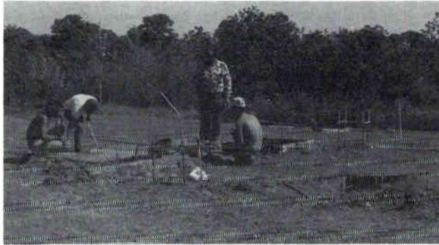
**12:22 PM/READY FOR CONCRETE.** . .Three concrete piers will be poured using 5.5 cubic yards of 3500 pound (2% calcium for quick-drying) concrete. 3,000 pounds of steel TVRO will sit here in six hours.
