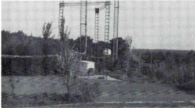
**10:59 AM/THE SITE.** . .Stakes in place, at 11 AM USTC will appear with a transit and locate the base center line. The terminal will go just behind the small tree left of center.
