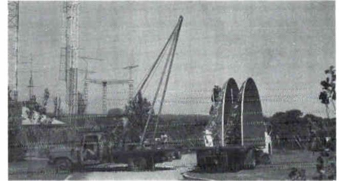
**1:33 PM/OFF LOADING TVRO.** . .Now the concrete is drying and the twin half-sections of the USTC SAT/FLECT I steel TVRO are off loaded from the lowboy trailer and placed into position adjacent to the poured base piers.
