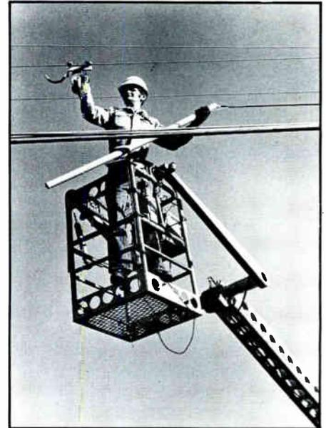
A member of Cablecom-General's construction crew strings a four-fiber optical cable from telephone pole to telephone pole in Joplin. The 3.56-mile aerial, fiberoptic cable replaces a conventional coaxial cable that carries video signals from the origination studio of Cablecom of Joplin/Webb City to the broadcasting tower on West 13th Street in Joplin. The smaller, lighter fiberoptic cable (attached to the pole held by the crewman) is easier to handle than the heavier coaxial cable seen below.
