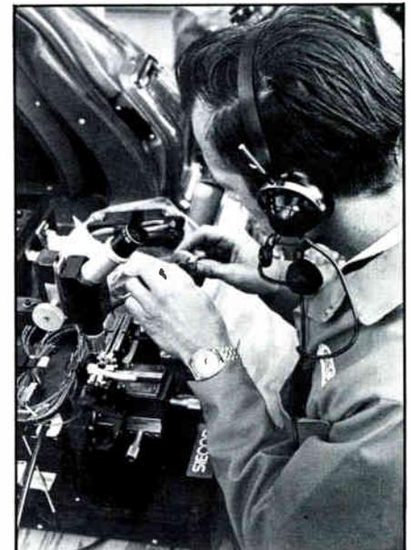
A technician prepares two lengths of fiberoptic cable for fusion splicing. The fusion splicer permits a technician to precisely align the tiny fibers and then to permanently join them in the field.
