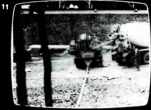
11. Pumper truck needed to get 152 cubic yards of concrete into foundations.
