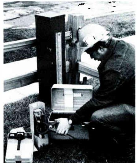
A G.E. Cablevision engineer uses the Dyna-Coupler™ to induce a tracing tone on an underground cable. This simple, clamp-like device combines the simplicity and speed of the traditional induction method with the accuracy of a direct electrical connection.
