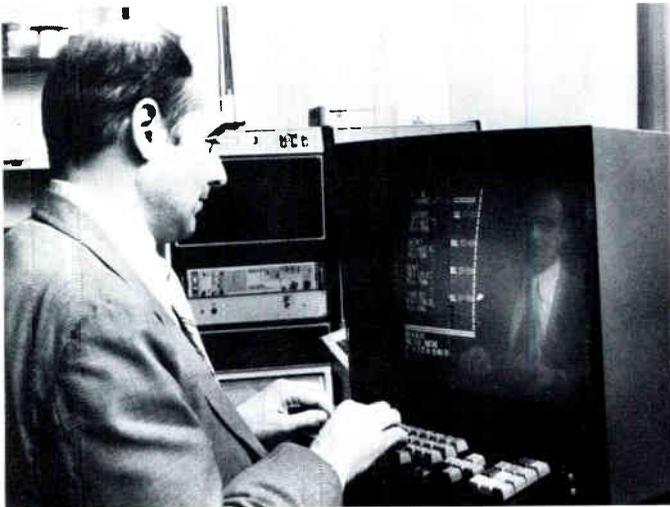
*Info-Text encoder is used by operator to set up all types of graphic material for the new "electronic newspaper" system, in color.*
