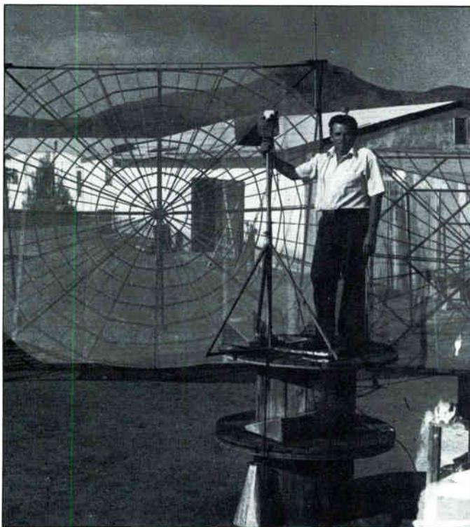
*Standing atop empty cable reels for support, spherical developer Oliver Swan with his unique feed horn developed for illuminating the spherical series antennas.*
