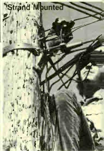
The new HS200, HS300 and HS400 Hybrid Splitters are built in the most unique housing on the market today! The quad mounted housing gives real flexibility to allow for strand or eave mounting, flush wall mounting, or horizontal mounting when drops are coming up from the floor or in cabinets when all the ports are needed to face down for real ease of installation.
