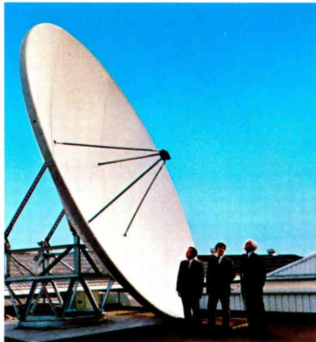
*Times officials examine new 7-meter satellite antenna at the company's Wallingford, CT headquarters plant. The TVRO is used for experiments and to test fiber optic satellite downlinks.*
