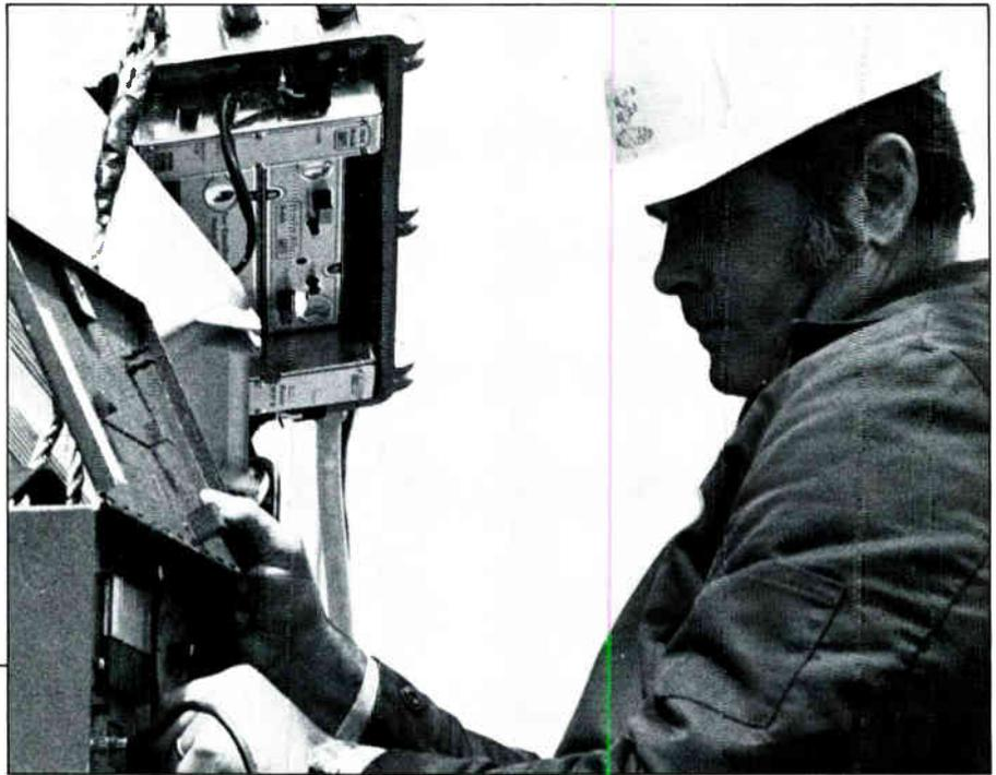
A Kingston Cablevision technician measuring interference at a feeder amplifier.
