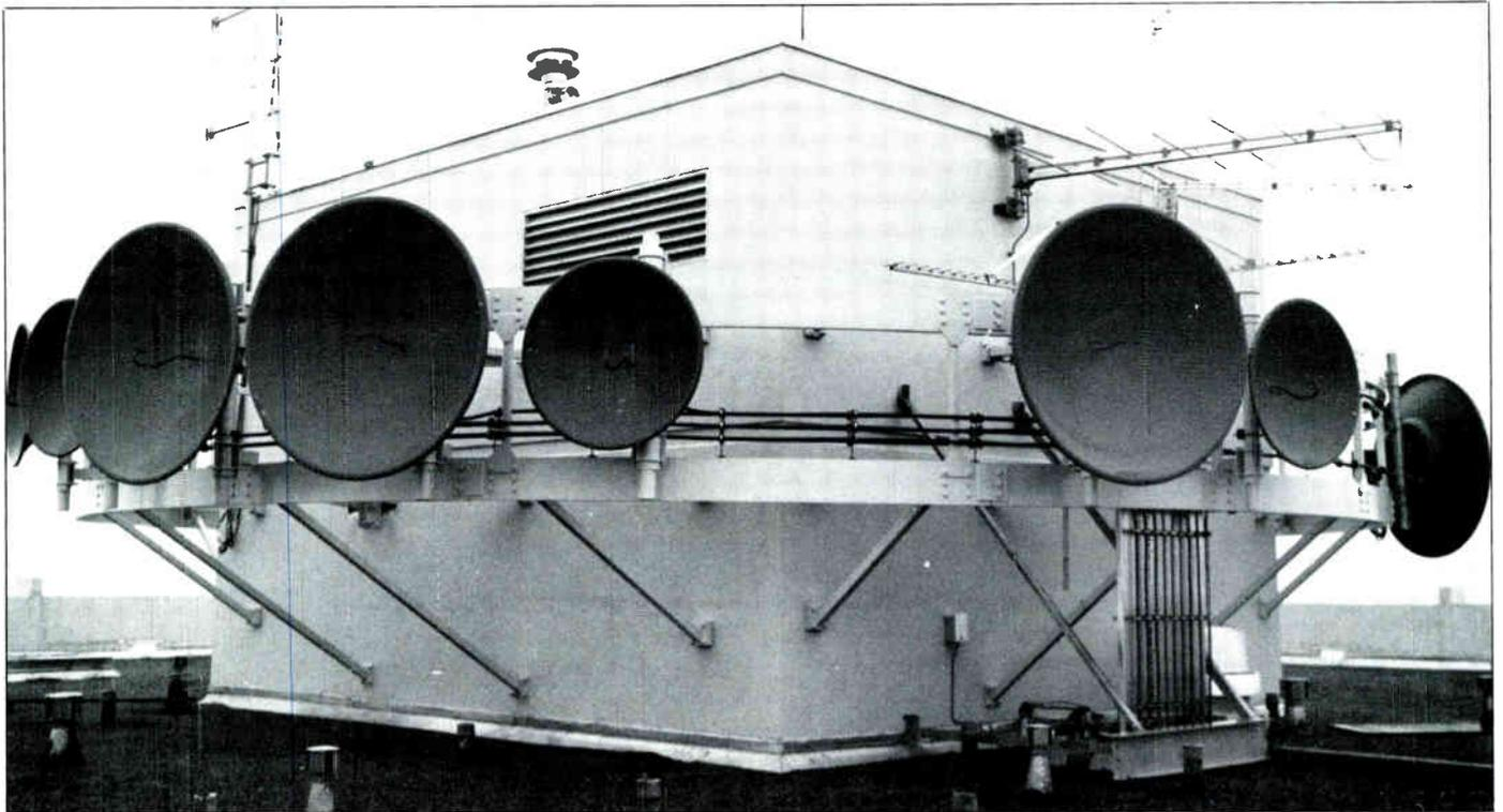
The MTC will use four-foot antennas to transmit in most directions and six-foot antennas to transmit to locations 18 miles away.
